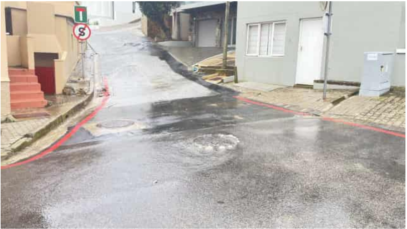
Photo 2: Surcharging Sewer Manhole Upstream of PS 1
