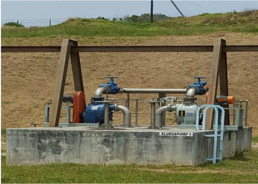
Fig 9: Sludge pump station
