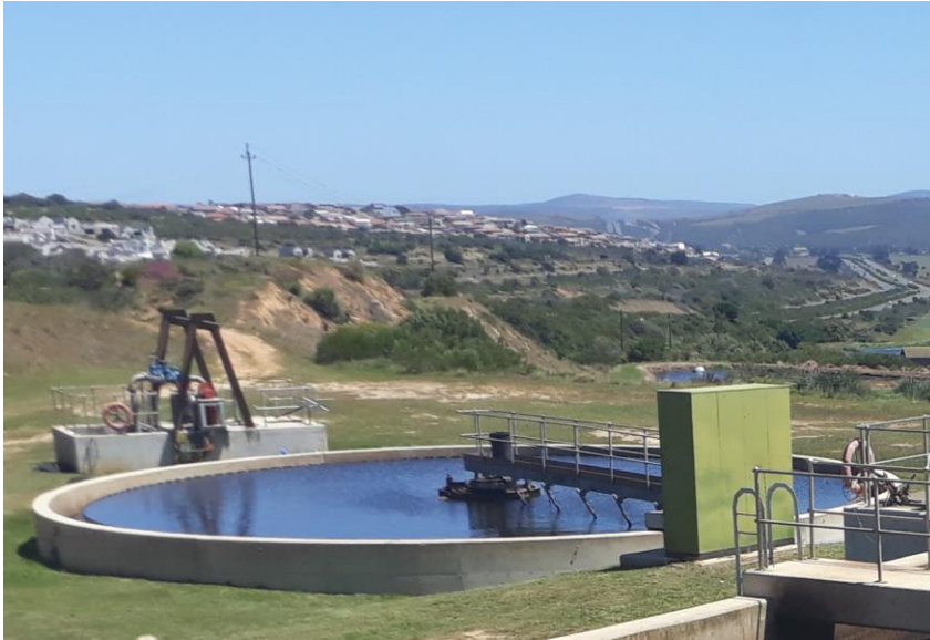
Fig 7: Existing secondary settling tank (SST)
