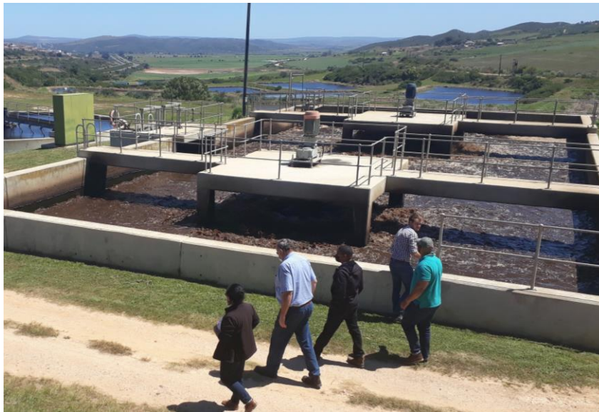
Fig 5: Existing reactor basin
